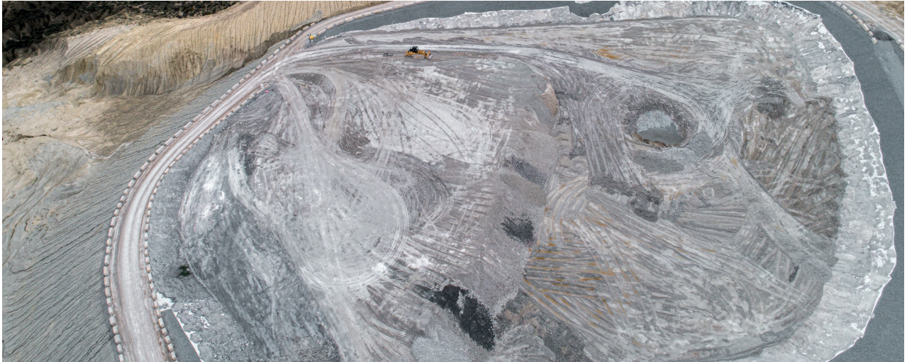
→ Cosentino® waste management plant
