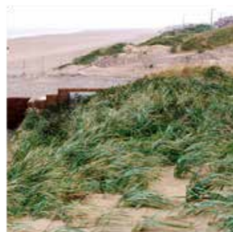
Marehalm vokset igennem GREENFIX Eromat for at undgå sanderosion.
