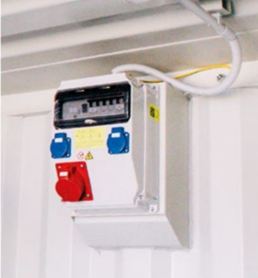
Distribution box with integrated sockets
