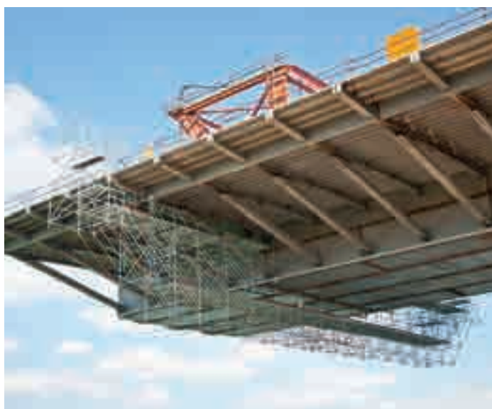
Thanks to the Allround bridging system, work scaffolding can also span even large distances free-standing, without the need for intermediate support for the scaffolding.
