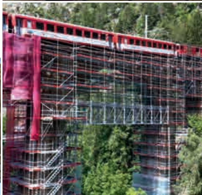
Thanks to the Allround bridging system, work scaffolding can also span even large distances free-standing, without the need for intermediate support for the scaffolding.
