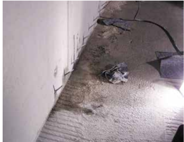
Construction Joint Injections
