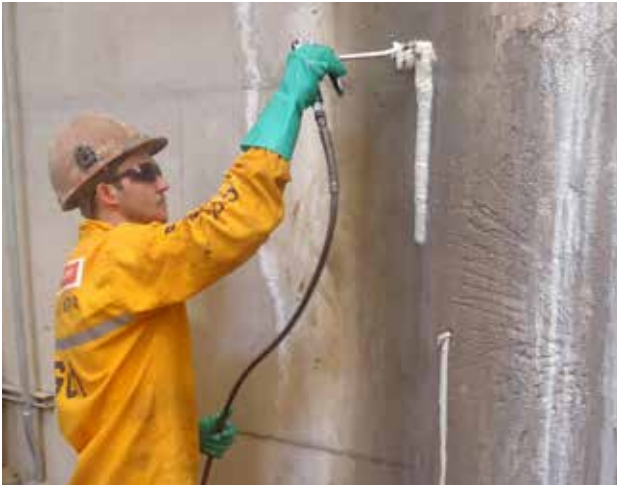
Crack Injections
