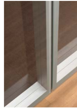
Flush bonded glazing
